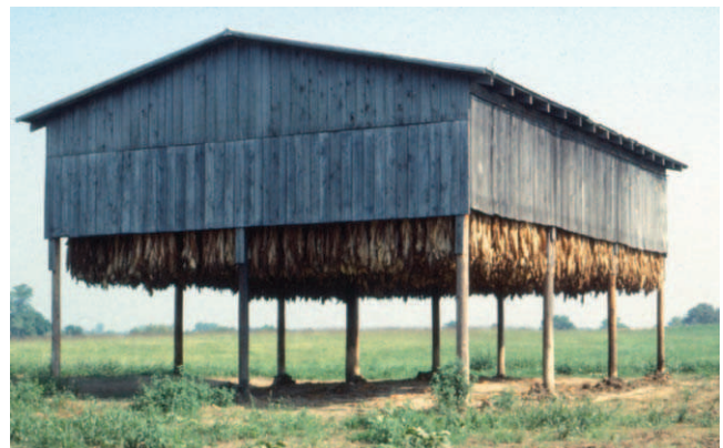
Figure 2. Economy barn of 2-tier height, 2 driveways with slip rails (not shown), partially enclosed side walls, and no doors.
