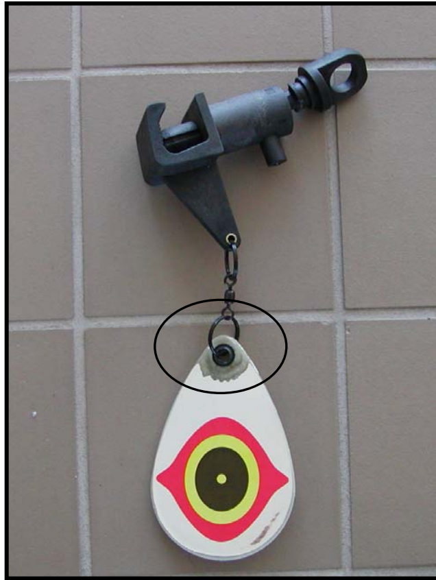
Figure 22. Corona-induced damage on diverter #5
