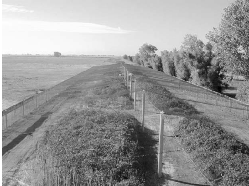
Fig. 2 Pen for controlled propagation of Riparian Brush rabbits measuring 162 m long, 30.5 m wide and with side fencing of 2.14 m in height. The top is covered with netting to prevent raptors from entering and the sides are covered with sheet metal (shown on the left ) but not yet installed on the right (photo by L.P. Hamilton)
