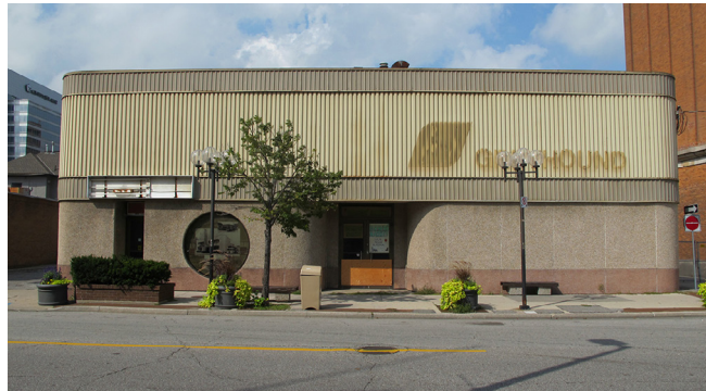
Existing South Depot Façade
