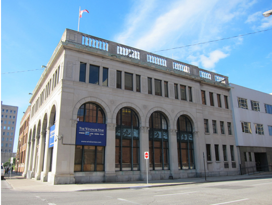
1927 and 1953 Windsor Star Building
