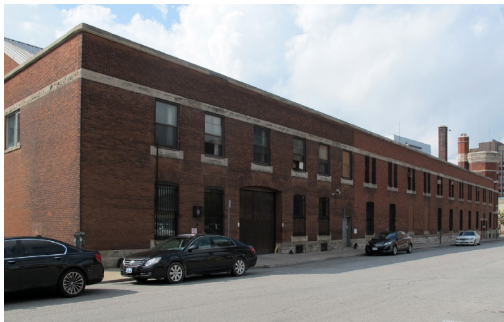
East Side at Freedom Way Looking North
